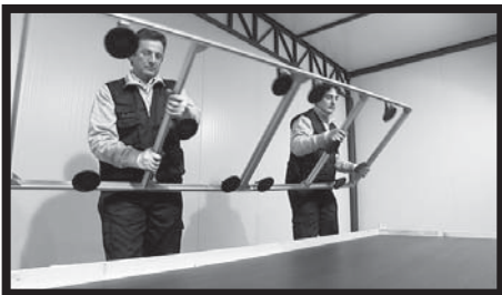
Fig.4/5 - All versions of KERLITE slabs, of size 300x100 cm, can be handled by two persons, using a special frame. Fix the frame to the slab when it is still on the pallet using the suction cups. Raise the frame and slab to eliminate the suction effect.
